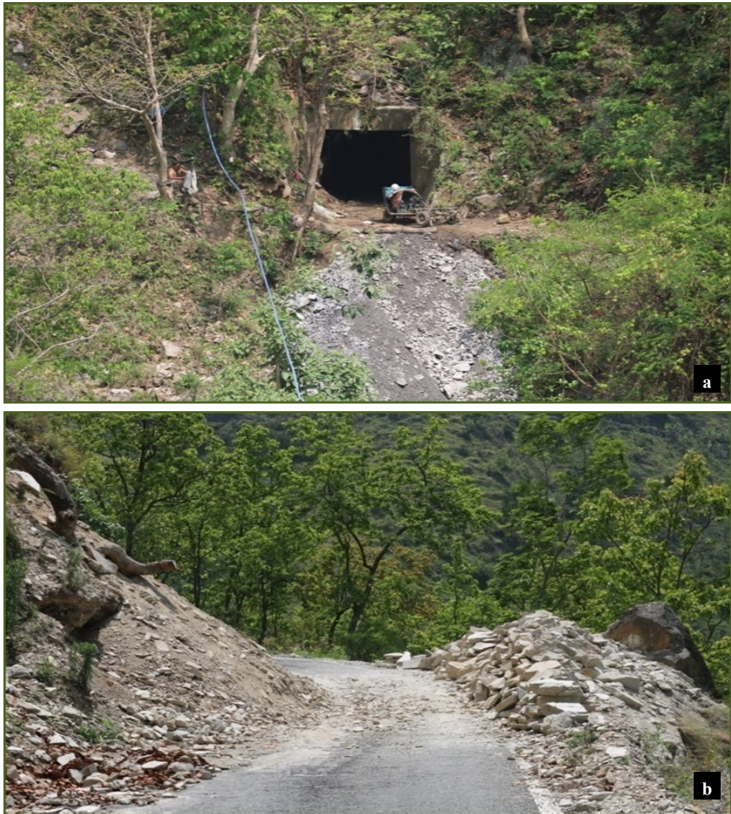
Figure 10. Human induced threat factors for the biodiversity, (a) tunneling and (b) frequent landslides due to current pre-dam construction activities at the Pancheshwar dam site, Central Himalaya.
