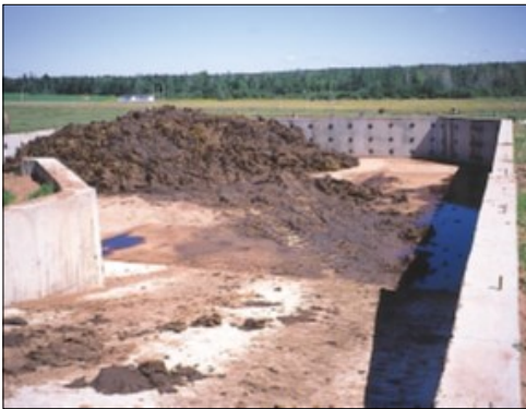
Figure 3.6. Solid or semi-solid manure storage - concrete slab with sidewalls and drive-in ramp.
