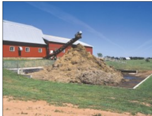
Figure 3.5. Solid manure storage - curbed concrete slab with ramp.
